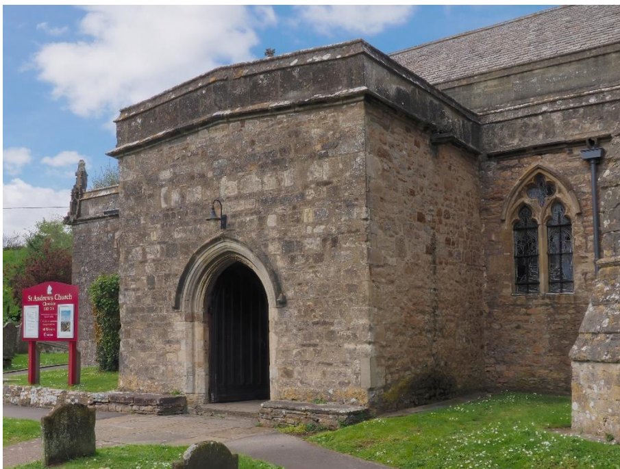
Figure 2 Exterior view of the Porch
